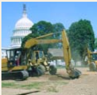
▲ Utility relocation work at the Capitol Visitor Center.
